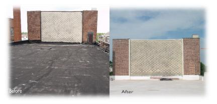
The beginning of safe, warm, and dry! One of the first things we had to do in order to keep water out of the theatre was repair the roof. Because it had been left in disrepair there was a large amount of rain being let in through the roof that damaged the interior of the theatre.
